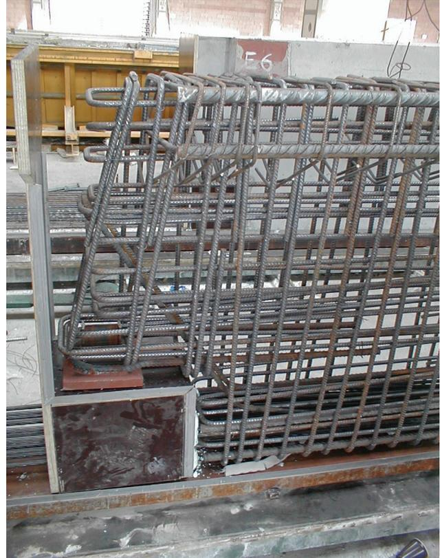
Fig. 35. Armature of the beam type “4000”
